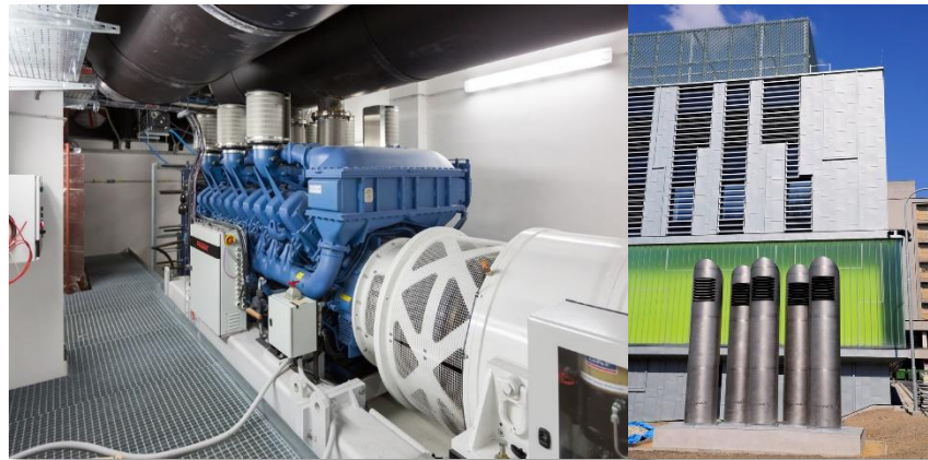
Dynamic rotating UPS 2x2,5MVA
